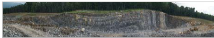
View of an impressive rock cut exposed during construction
