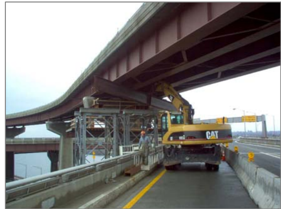
Erection of Mabey Towers (GPI design)
