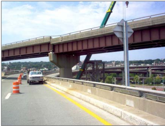
Erection of Mabey Towers (GPI design)
