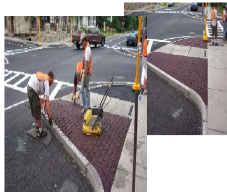
Stamping Asphalt in Wallingford
