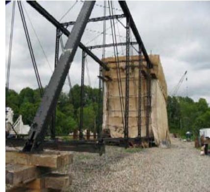
Maidstone Bridge Containment
