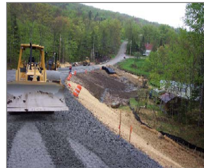
Subbase application in Winhall
