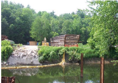
Gorman River Bridge
