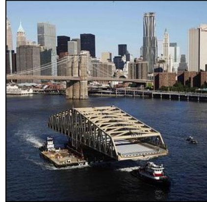
The new 300-plus-foot swing drawbridge arrived atop two barges
