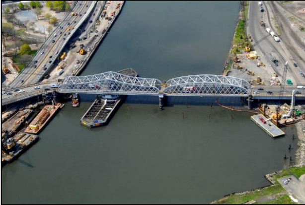
The Willis Avenue Bridge pre-construction
